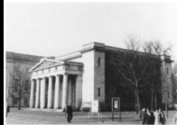
Fig. 5. Three views of the Royal Guard House from the southeast (photos: author).
